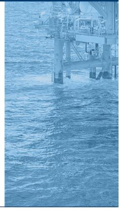
Offshore oil platforms rely on caissons, or columns of steel, to serve as a critical part of their operation. Caissons house and protect equipment, such as seawater pumps and piping. These vital components are highly susceptible to corrosion and degradation as they extend into the splash zone and may be submerged in the ocean. A major oil company operating on the Gulf Coast needed to find proper treatment that could extend the lifespan of this critical equipment and avoid excessive downtime.
